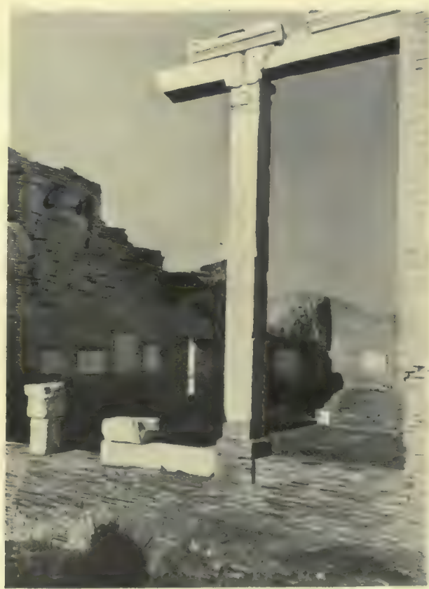
4. Room G, from Southeast.
